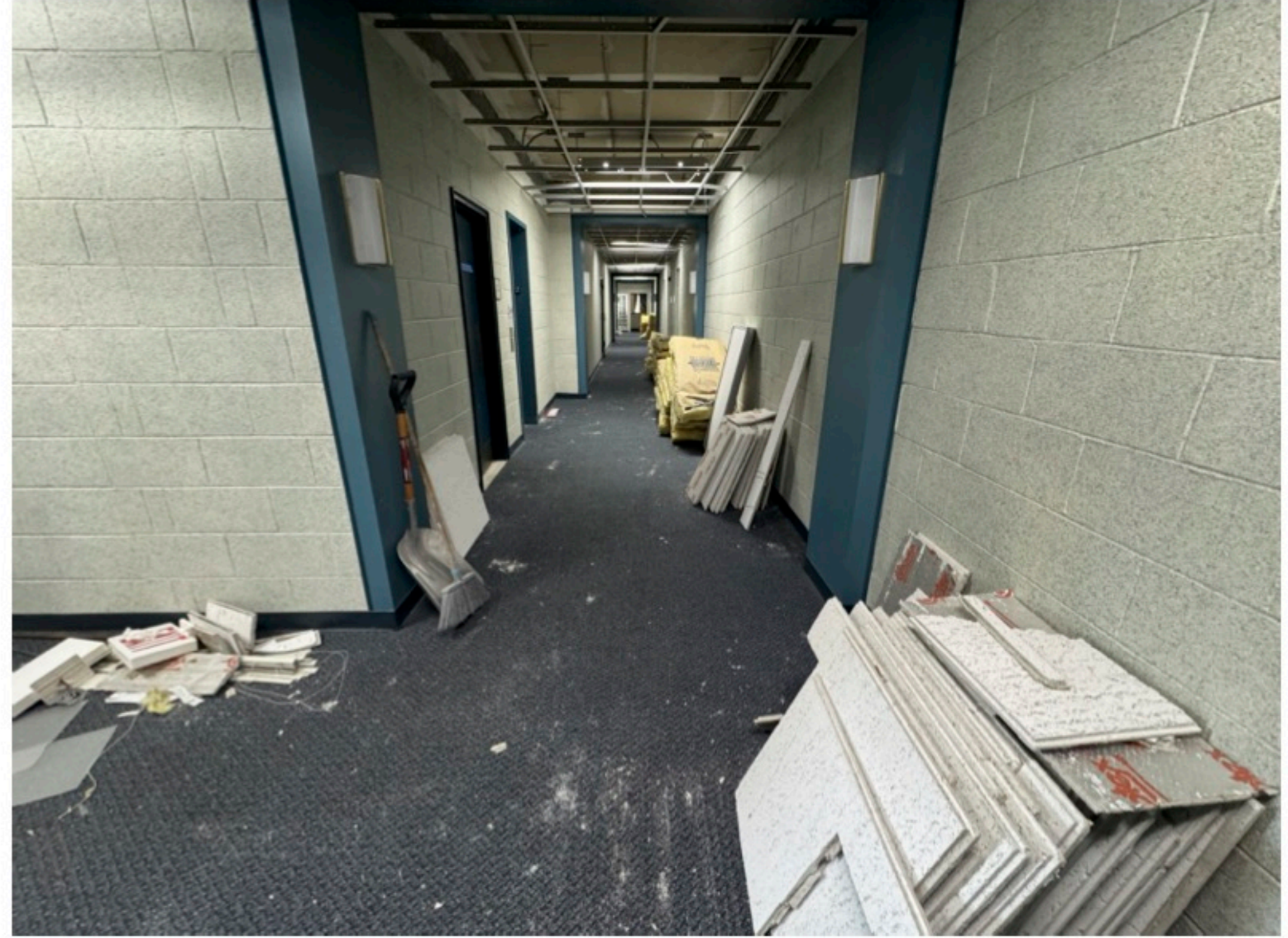
Ceiling demo. at 2nd floor of Ed. Bldg.
