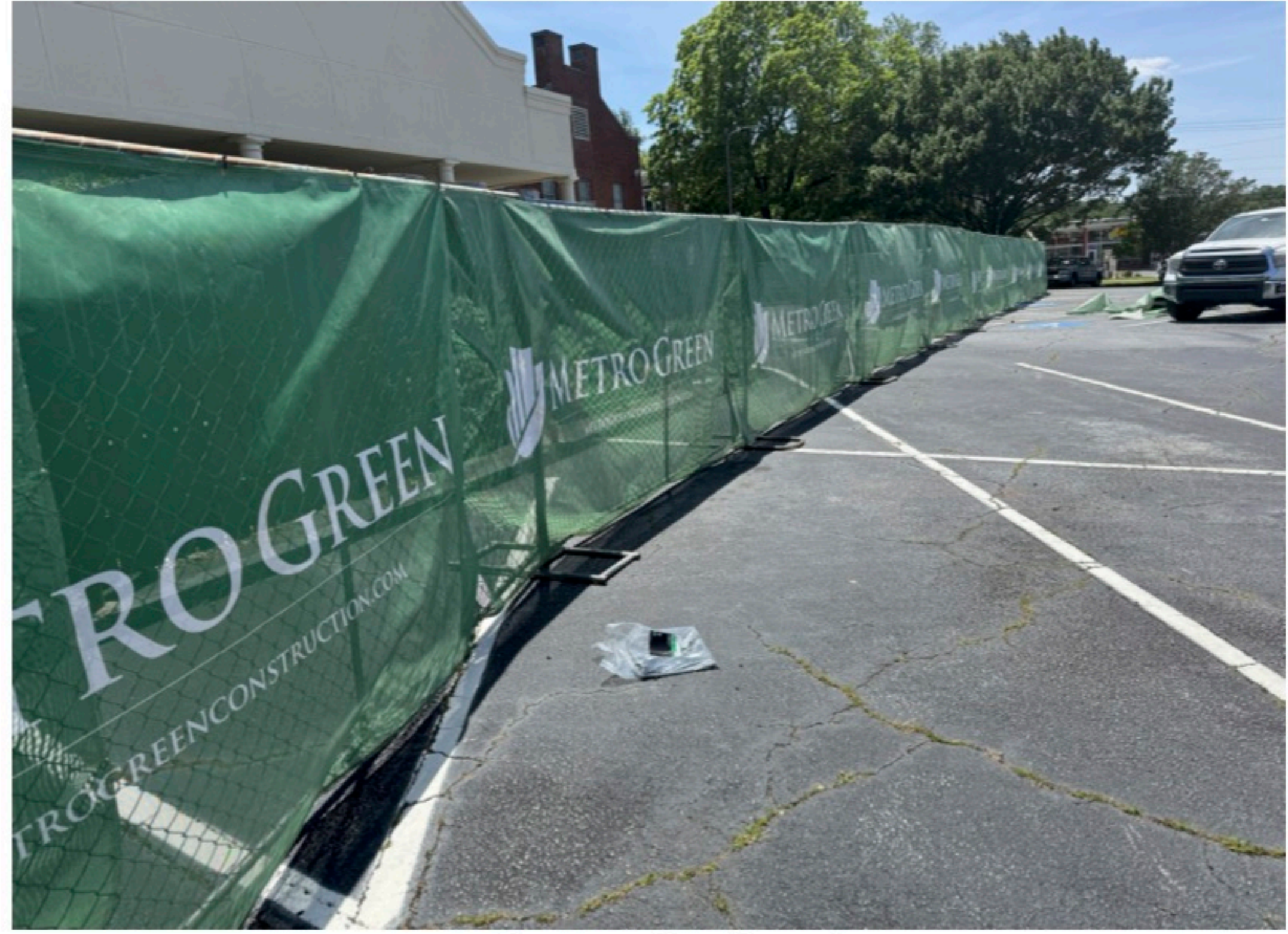
Construction fencing for demolition
