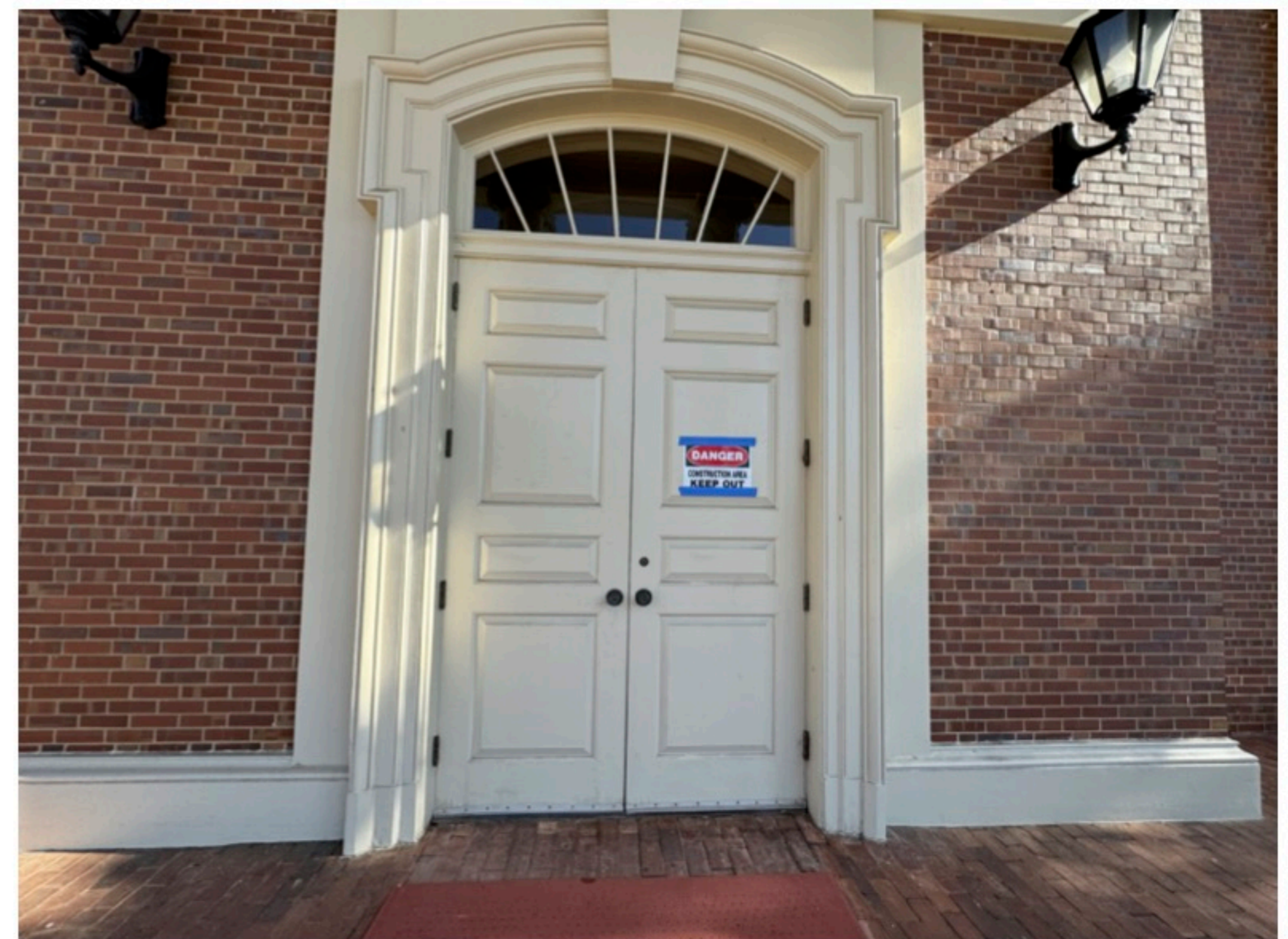
Safety signage added to construction site (all doors)
