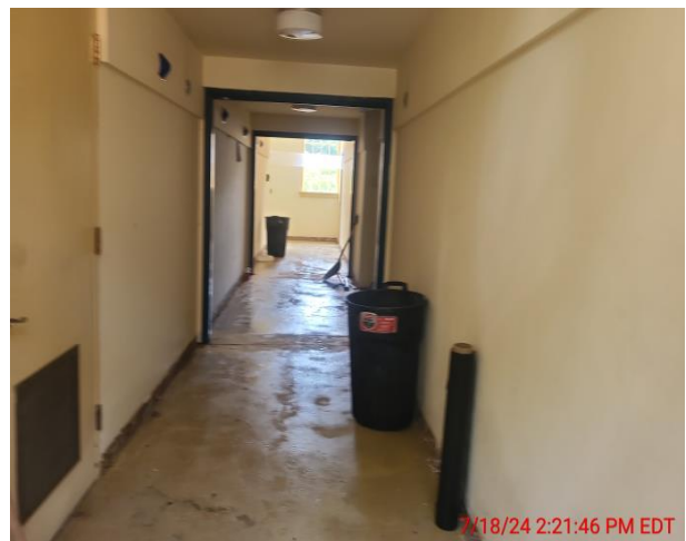
Mastic abatementment after carpet removal.
